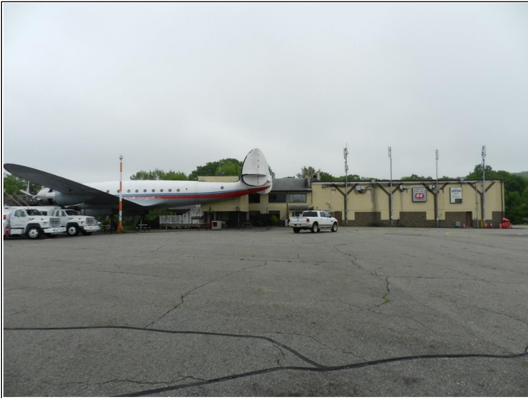
Figure 4-11. Poles Penetrating the Part 77 Transitional Surface Adjacent to Administration Building
