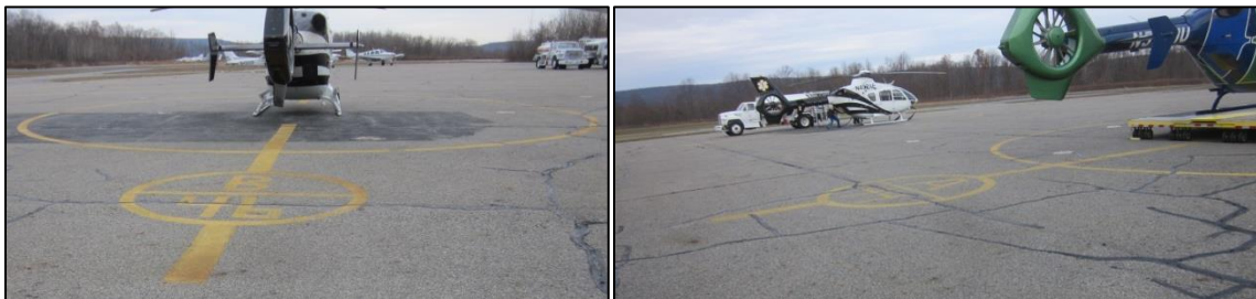
Figure 3-18. Existing Helipad Identification Markings
