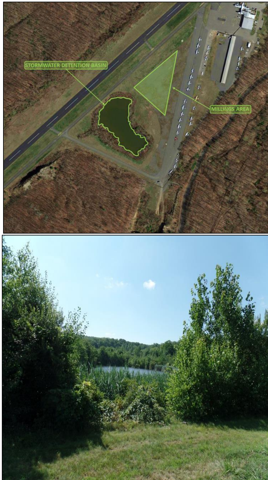
Figure 1-20. Stormwater Detention Basin and Milling Area
