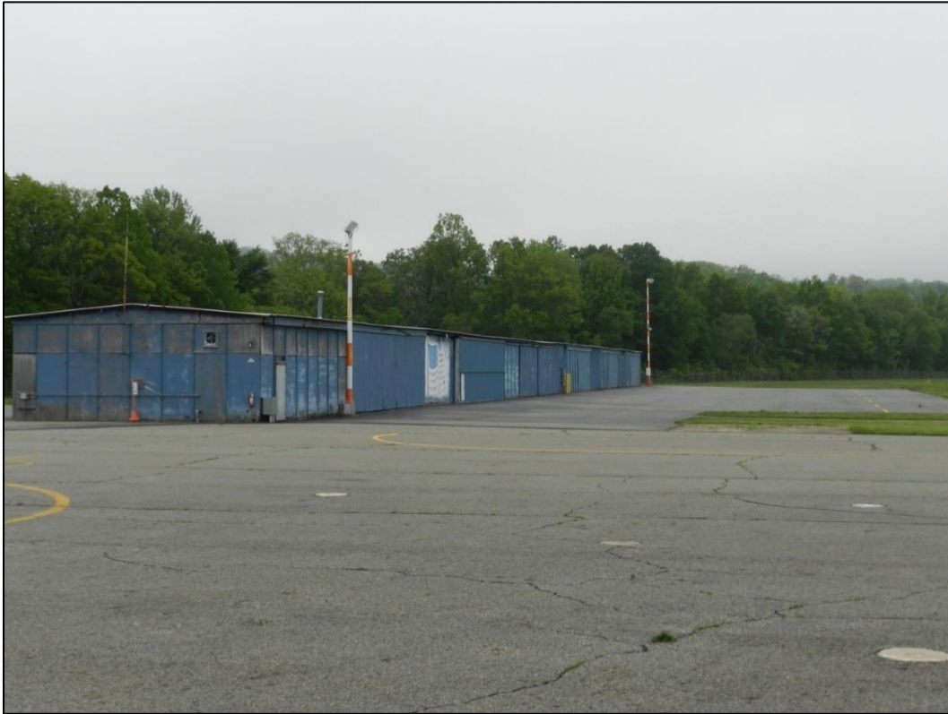
Figure 4-12. Poles Adjacent to T-Hangar that Penetrate the Part 77 Transitional Surface
