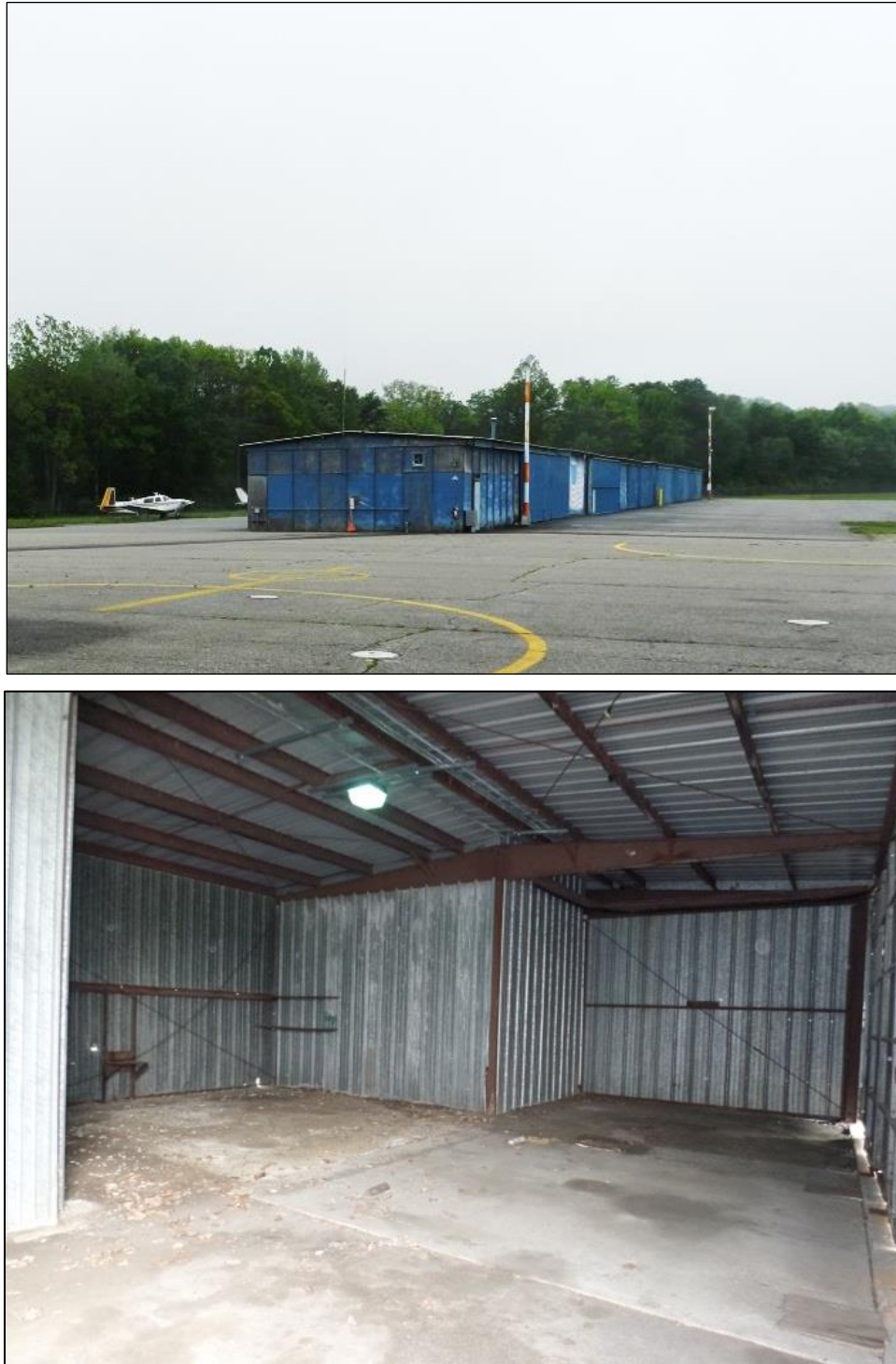
Figure 1-13. Exterior and Interior of the T-Hangar
