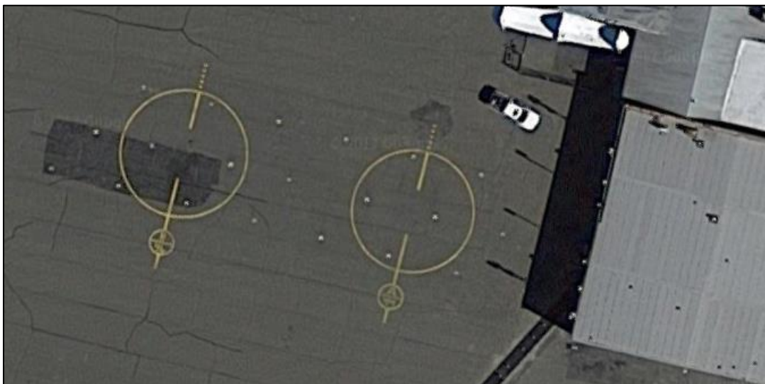
Figure 3-17. Existing Helicopter Pads
