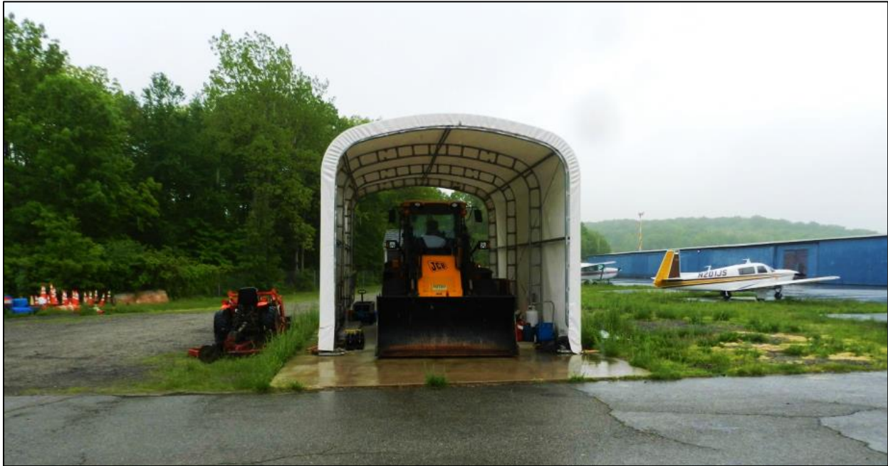
Figure 1-18. Front-end Loader Snowplow
