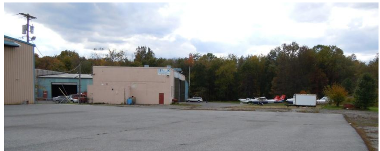
Figure 1-13: Aircraft Maintenance with apron access
