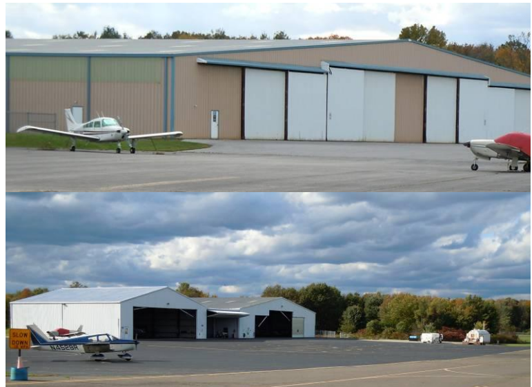
Figure 1-12: Community Hangars #1 (top) and #2 to #4 (bottom)
