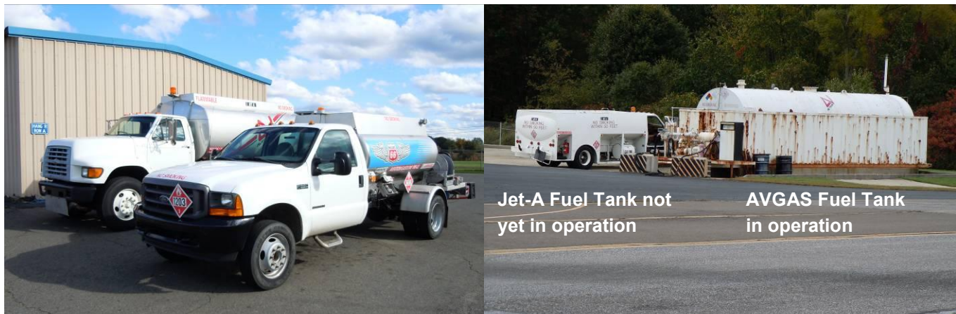
Figure 1-17: Fuel Trucks (left); Fuel Tanks (right)
