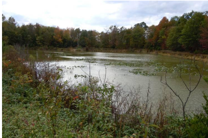
Figure 1-20: Stormwater Detention Pond
